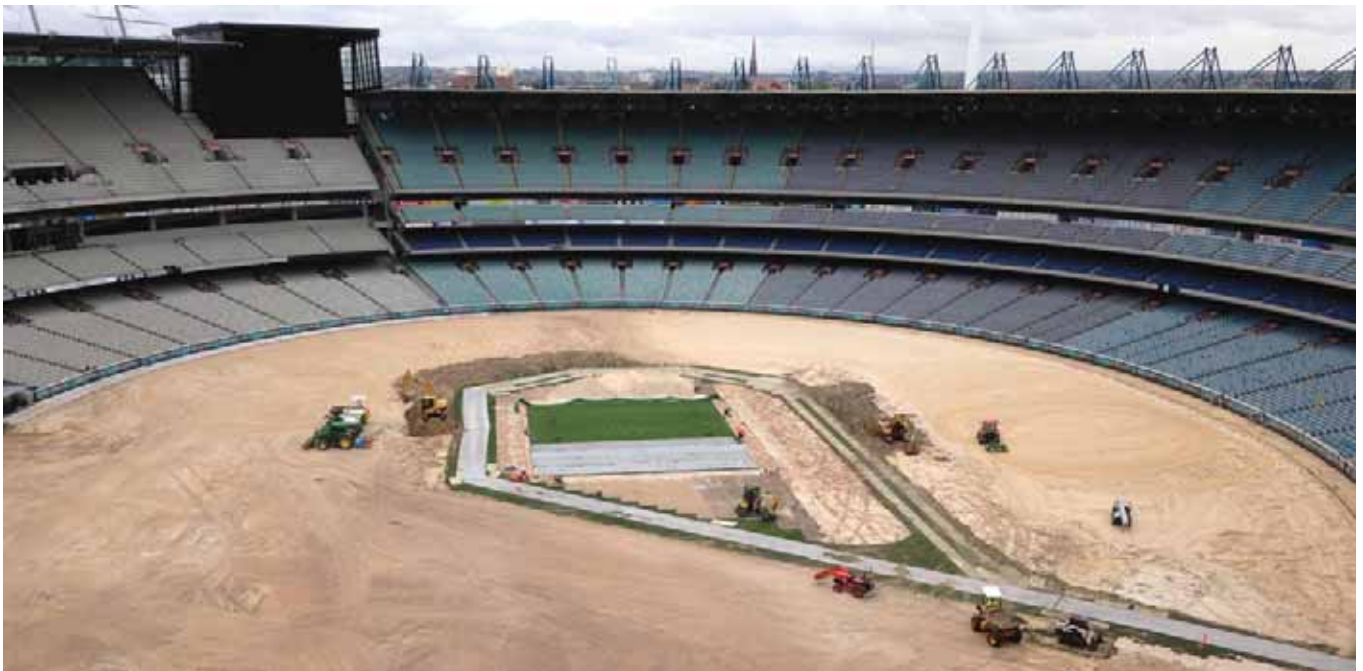
The entire MCG turf surface was replaced immediately after the 2014 AFL season.
